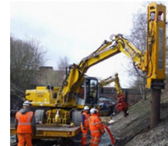
The main disadvantage of gravity pads was that the production and transportation of large amounts of concrete for them contribute to higher carbon emissions. Across the TAM project area 828 concrete pad foundations were removed from the design plan and converted to CHS piles, saving 2,630kg CO<sub>2</sub>e per location and 2,219,040 Kg CO<sub>2</sub>e in total. Furthermore, it generated construction efficiencies and reduced time on site.
