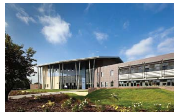
Penyrheol Comprehensive School Rebuild Project – CEW Demo 2009
