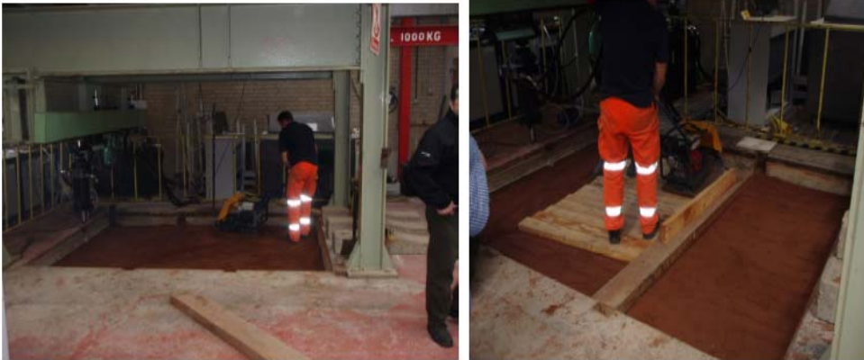
Figures 2: Materials Installation
