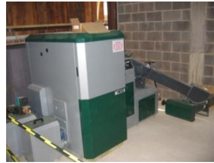
Biomass Wood-fuelled boilers
