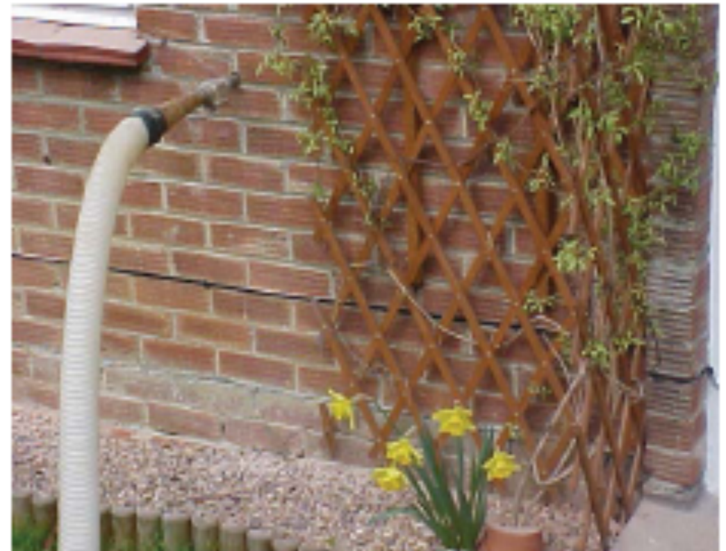
Figure 12: Insulation being injected into the wall
