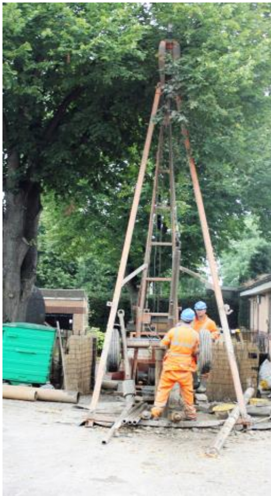
Borehole drilling and development
