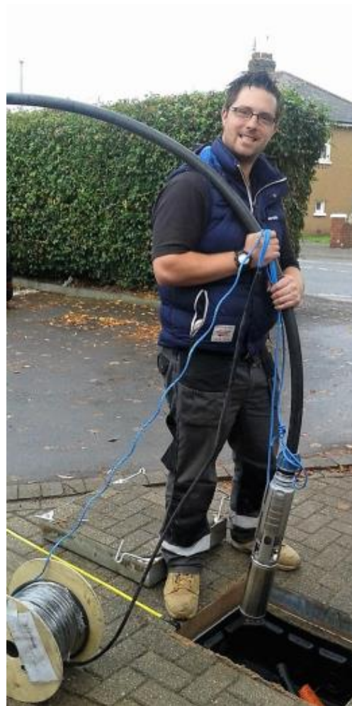
Borehole pump installation
