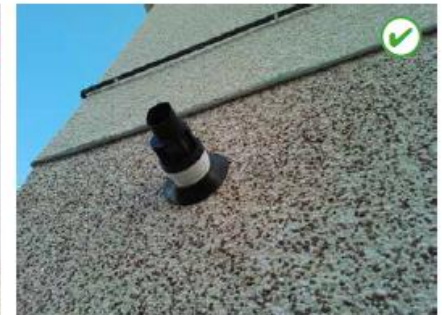
Figure 37: sealed penetration (good practice)
