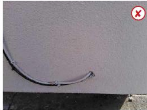
Figure 38 - cable clipped
