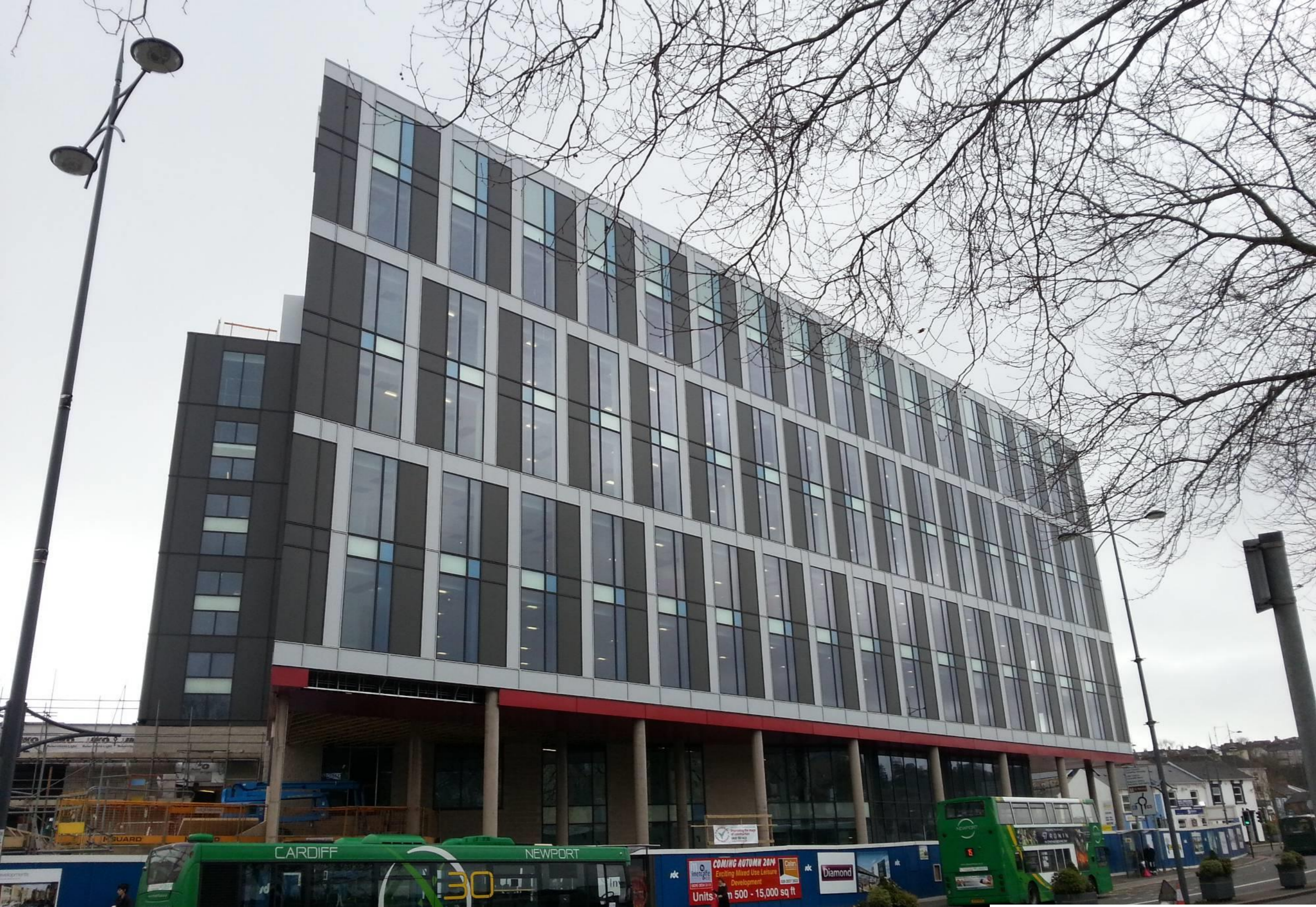
March 2014 – Nearing completion...
