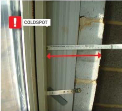
NO OVERLAP OF WINDOW AND CAVITY
