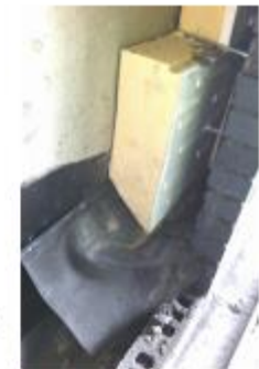
CUT INSULATION AROUND CAVITY TRAY
